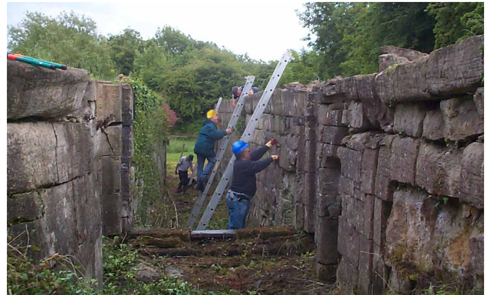
LADDER WORK AT LOCK 1 — June 2003 *****
