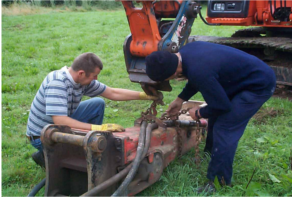
THE HYDRAULIC BREAKER BEING PREPARED FOR USE
