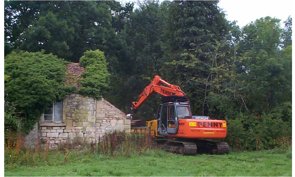
A "SERIOUS PIECE OF KIT" BACKS INTO CAISSON FIELD — August 2003
