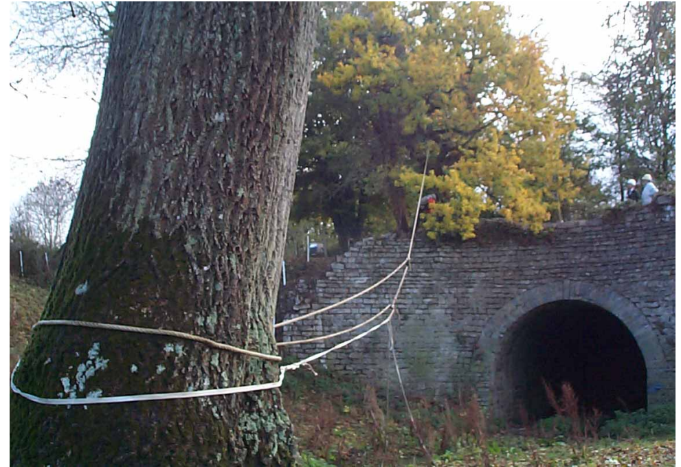
ROPES AND PULLEYS TO PULL THE FALLING TREE IN THE RIGHT DIRECTION
