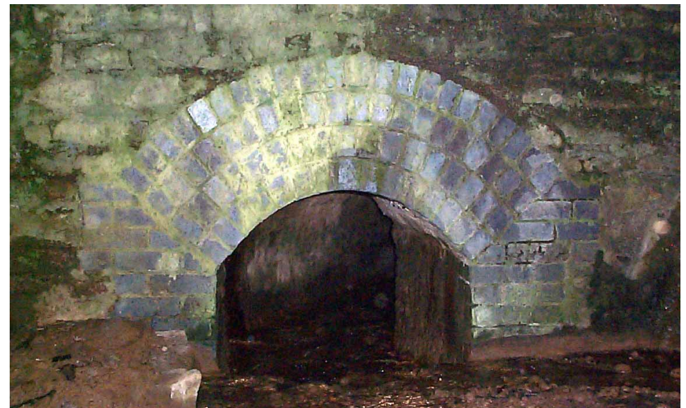
INSIDE THE AQUEDUCT ARCH THE CULVERT UNDER THE RAILWAY EMBANKMENT
