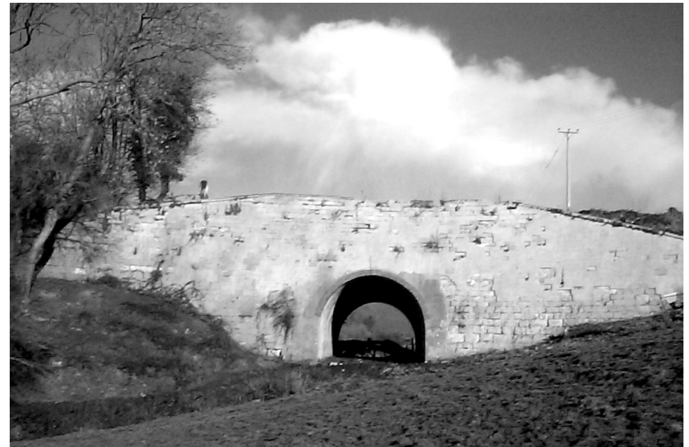
DUNKERTON 'BIG' AQUEDUCT AT SEVERCOMBE — December 2000
