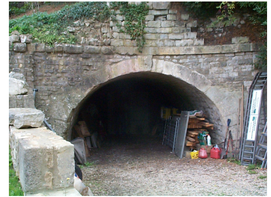
WELLOW TUNNEL NORTHERN PORTAL Restored by the owner
