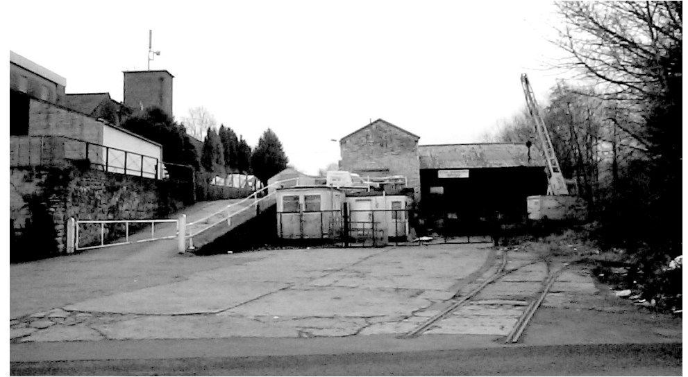
DISUSED SIDING AND OLD COLLIERY BUILDINGS AT LUDLOW'S PIT, RADSTOCK
