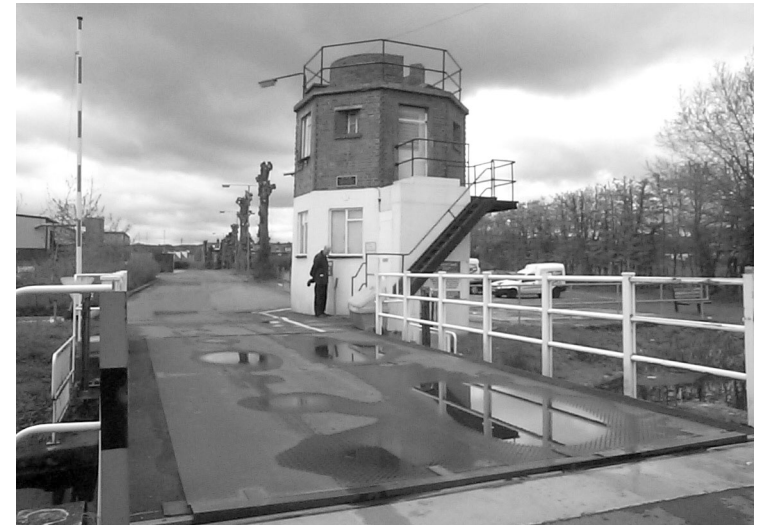
Above: NEW AND OLD AT BONDS MILL High-tech electro-hydraulic lifting bridge, constructed with modern plastics, contrasts with a wartime relic.
