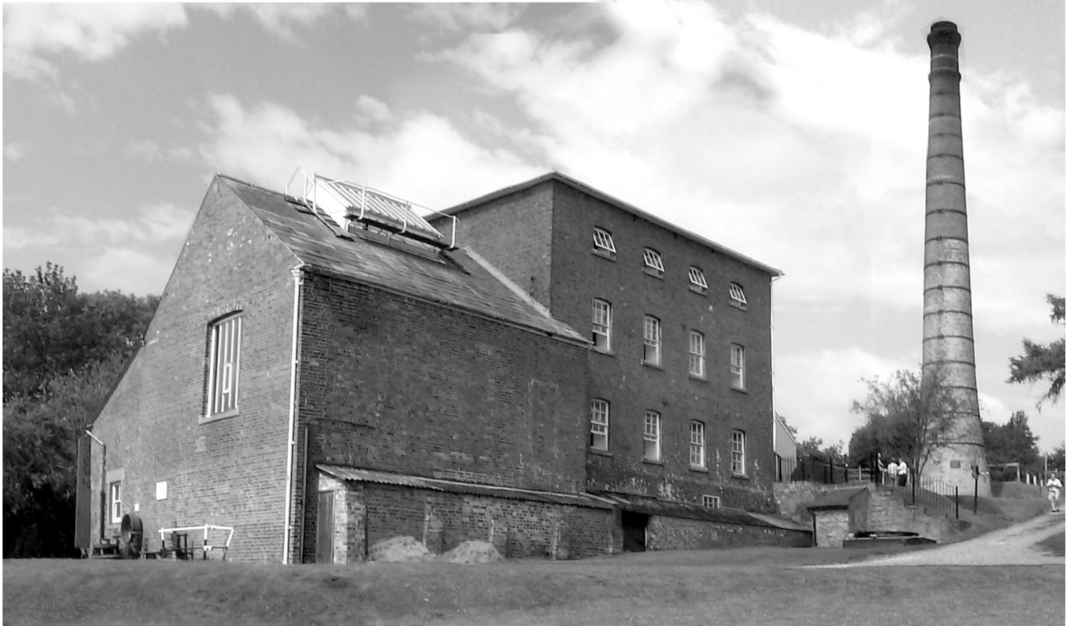
CROFTON PUMPING ENGINE - K & A Canal, Great Bedwyn — July 2004 From left to right: Boiler house, Engine House, Flues (low lean-to), Chimney.
