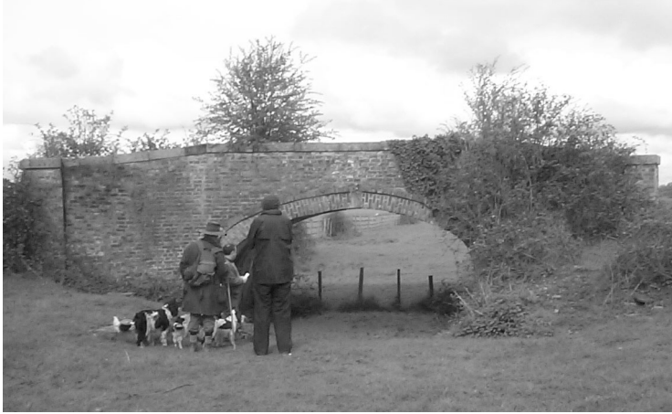
WESTFIELD BRIDGE — The only trace of the canal at this point, now left standing forlornly in a field. The lock is buried beneath the grass.
