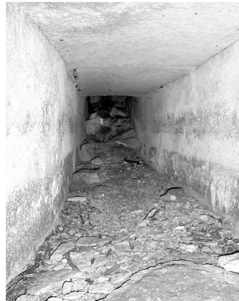
INSIDE THE SLUICE OF LOCK 5 — May 2004
