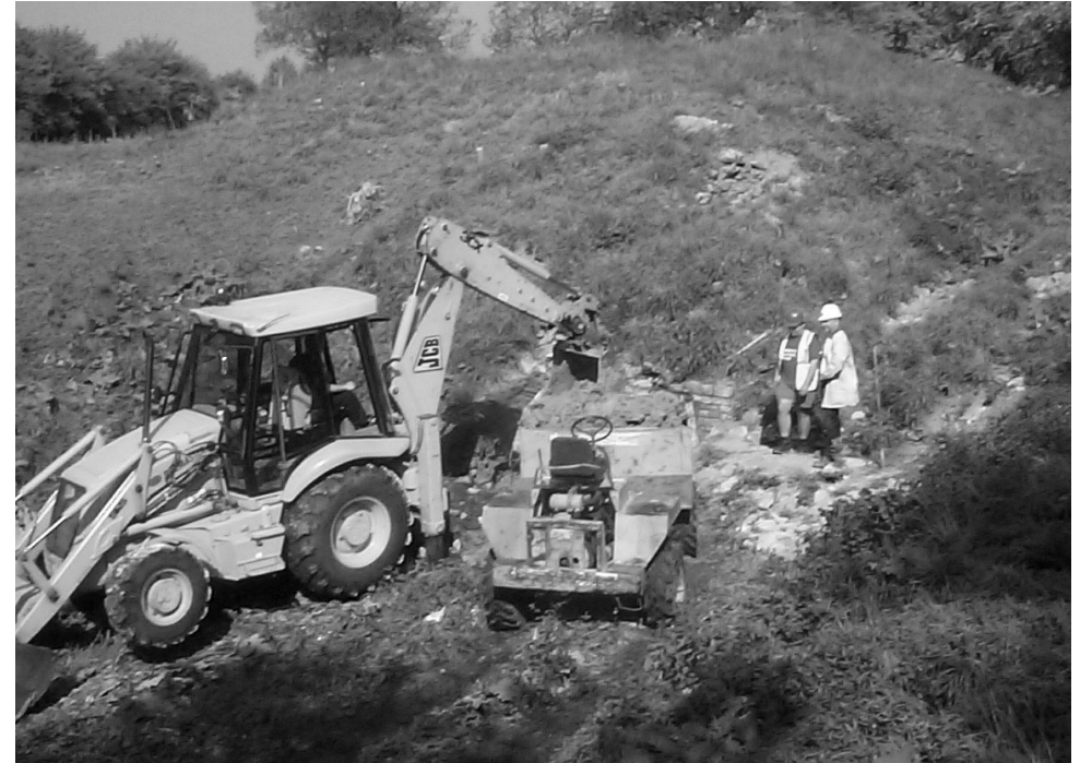
THE EXCAVATION GETS UNDER WAY — May 2004
