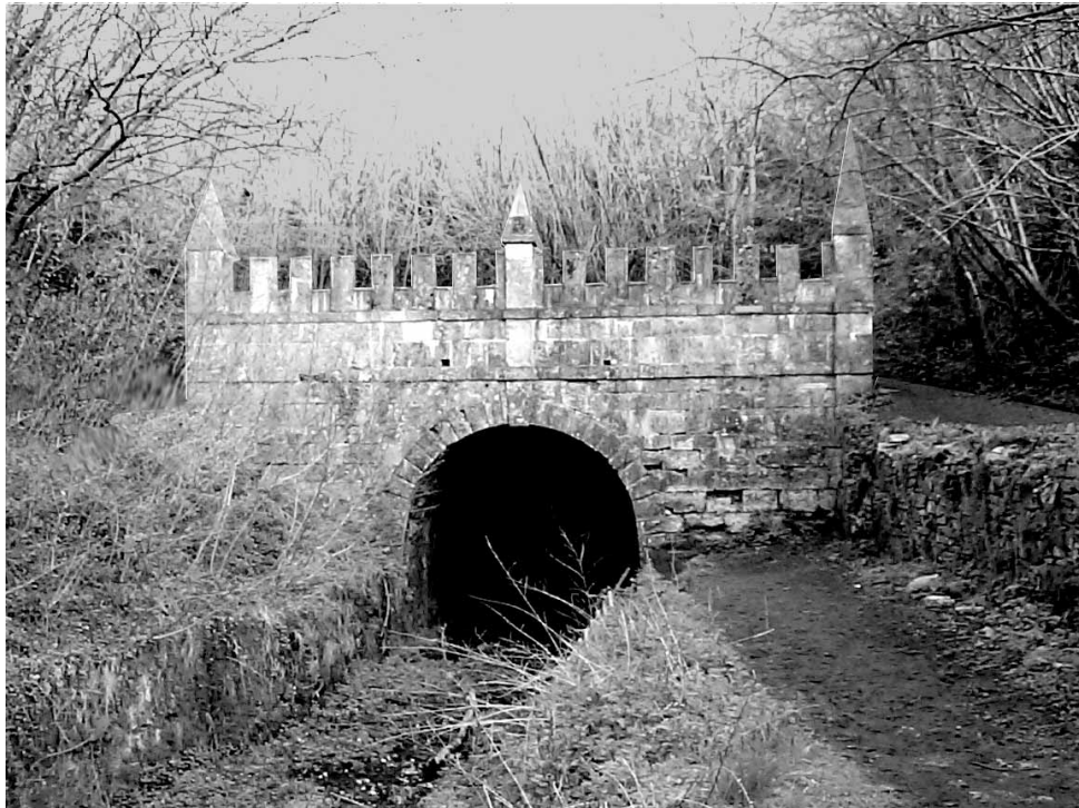
THE RESTORED PORTAL OF SAPPERTON TUNNEL
