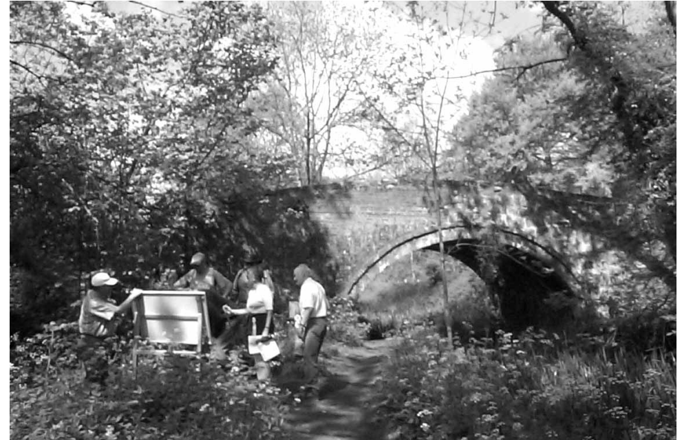
WHITEHALL BRIDGE NEAR TRILLIS — May 2004
