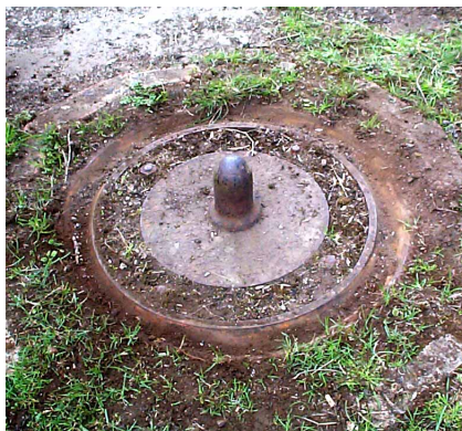
THE ORIGINAL BEARING RING AND PINTLE OF THE SWIVEL BRIDGE
