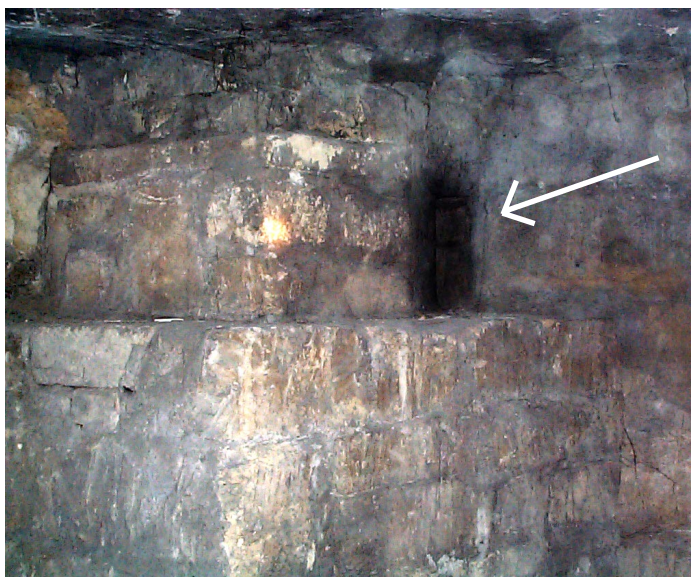
THE TOP OF THE HOLE IN A PLINTH SEVERAL FEET ABOVE CELLAR FLOOR LEVEL
