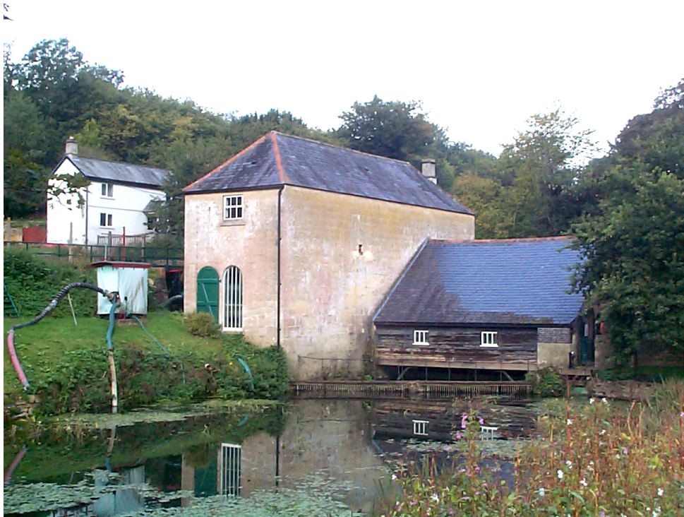
AN EXTERIOR VIEW OF CLAVERTON PUMP HOUSE
