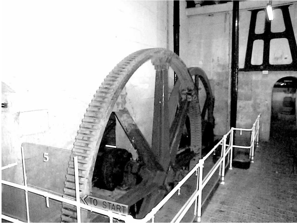
THE PIT WHEEL (nearest) DRIVING THE FLYWHEEL AND CONNECTING RODS
