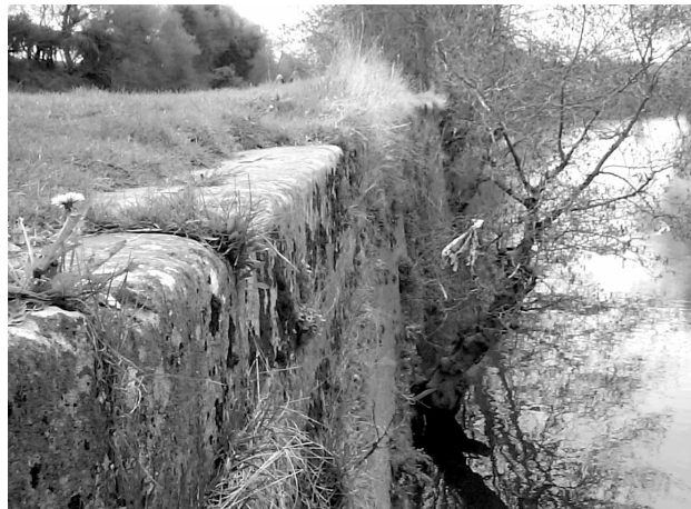
COPING STONES OF LONDONDERRY WHARF STILL VISIBLE (April 2006)
