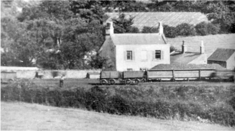
DRAMWAY WAGGONS —A view from the west of the Dramway depot at the Bath-Bristol Road Crossing around 1900, showing several of the front-tipping wagons from California Colliery waiting on the sidings.
