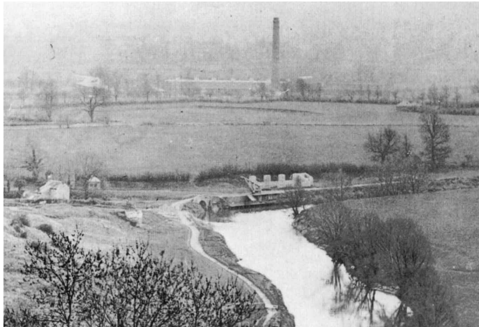
LONDONDERRY WHARF from the north around 1900. — The coal storage bunkers, crane and coal chute can be seen on the wharf, together with the small weigh bridge house to the left. In the distance can be seen the chimney of the Polysulphin Works opposite Avon Wharf.
