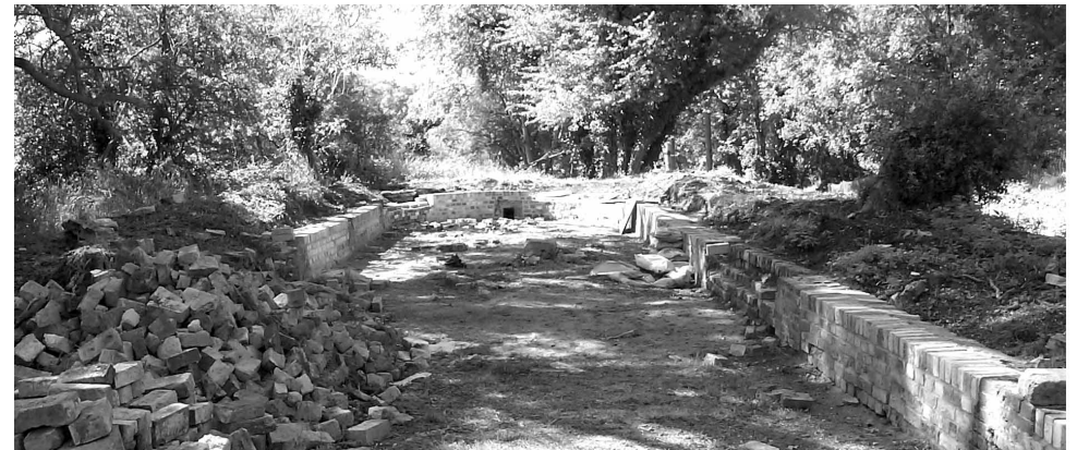
THE DRY DOCK in the process of rebuilding
