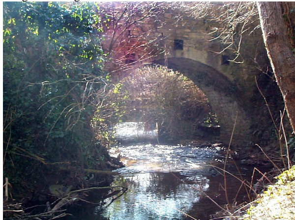
THE WIDENED TRAMWAY BRIDGE AT OLD WELTON PIT
