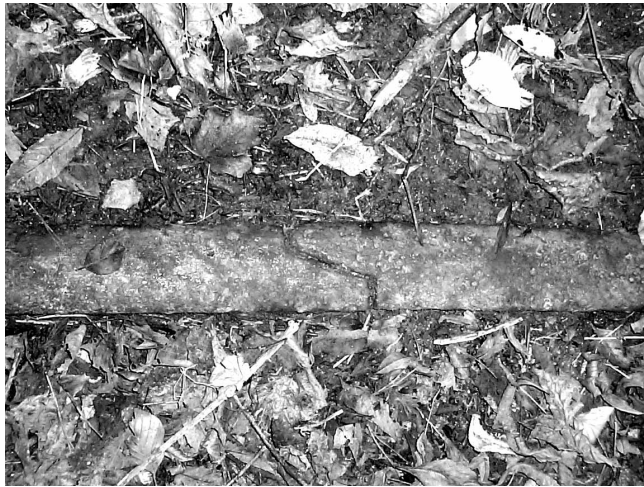
A MURHILL RAIL, STILL IN SITU - Showing the overlapped joint
