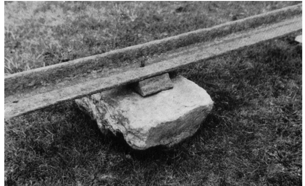
WROUGHT IRON RAIL, CHAIR AND STONE SLEEPER BLOCK
