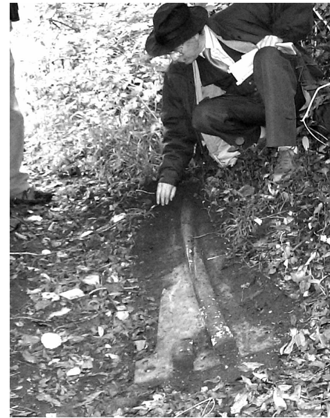
MIKE CHAPMAN EXAMINING A SECTION OF THE MURHILL RAIL WHICH FORMED PART OF A SET OF POINTS
