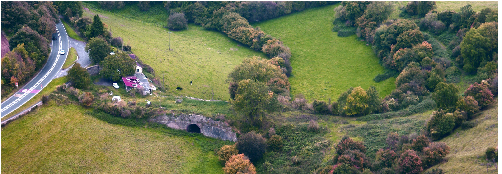
Below: AERIAL VIEW OF DUNKERTON AQUEDUCT
