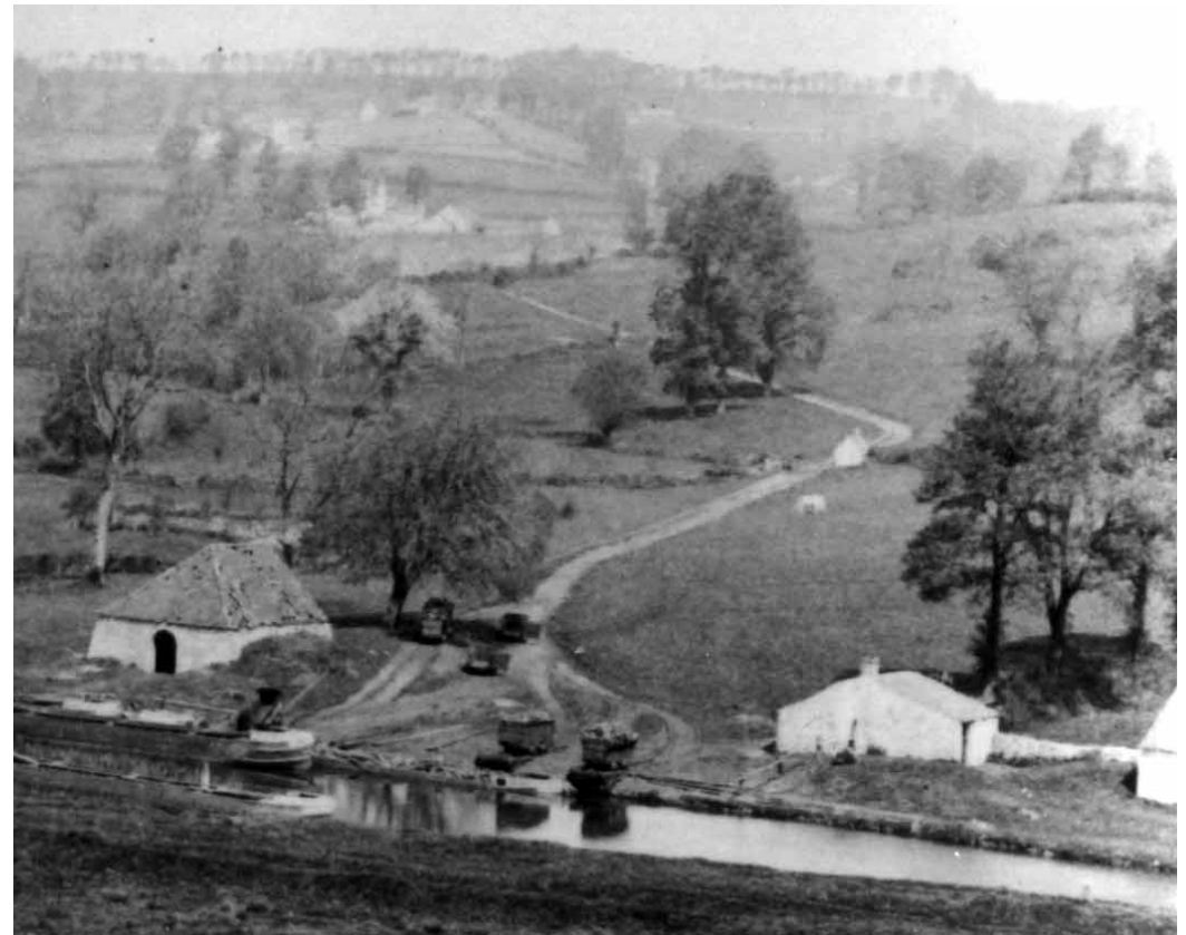
Loaded waggons can be seen waiting on staites, ready to tip their contents directly into the boats.
