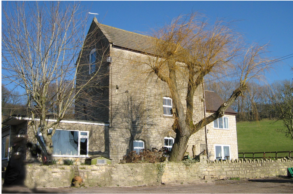
HEYSWOOD COLLIERY PUMPING ENGINE HOUSE
