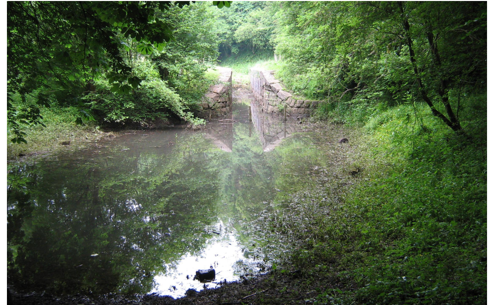
THE POND BELOW LOCK 15 IN WATER FOR THE FIRST TIME IN EIGHT YEARS
