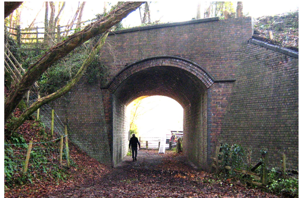
THE RAILWAY BRIDGE BELOW LOCK 15
