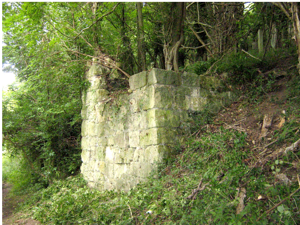
The masonry platform near Lock 19
