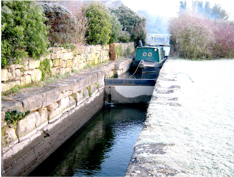
THE ENTRANCE LOCK AT DUNDAS — March 2009 Showing the middle gate closed to hold back the waters of the K & A Canal during maintenance work on the S.C.C.
