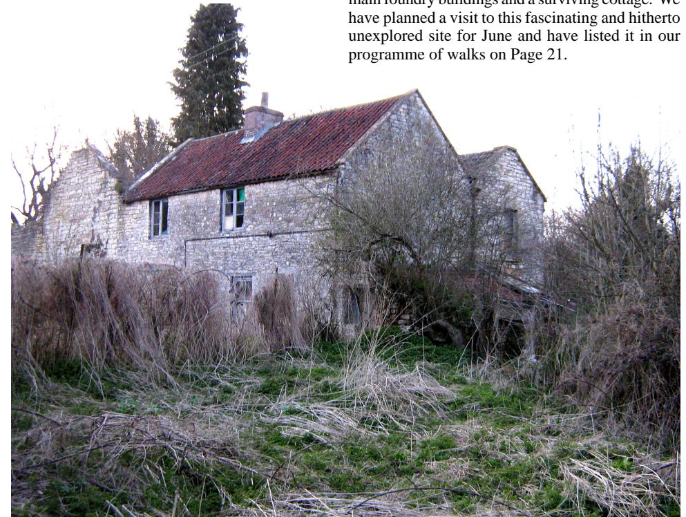
BUILDINGS ON THE PAULTON FOUNDRY SITE — April 2010
