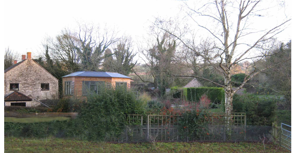
PAULTON FOUNDRY SITE —December 2010 The cottage is the only remaining landmark visible from this viewpoint
