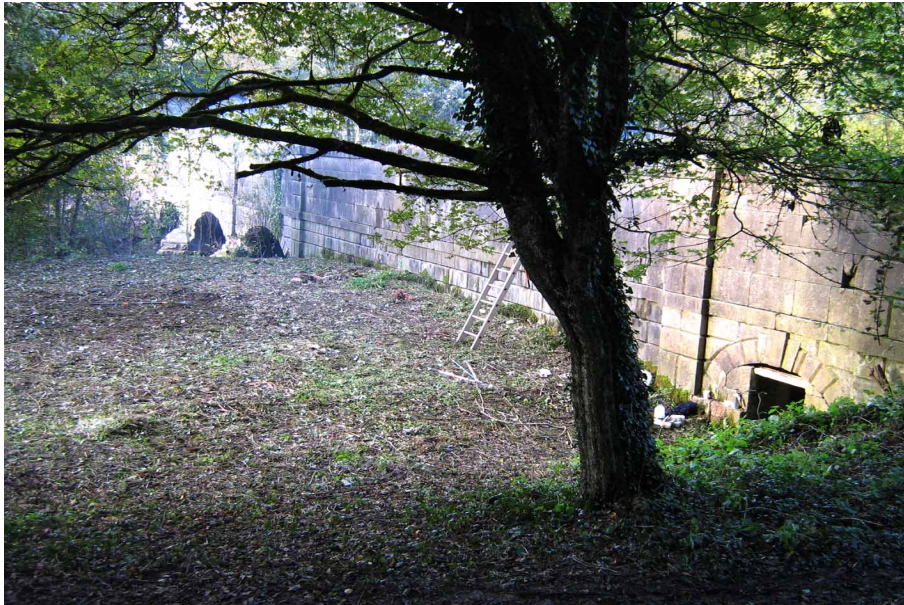
MURTRY AQUEDUCT AFTER CLEARANCE WORK — October 2010
