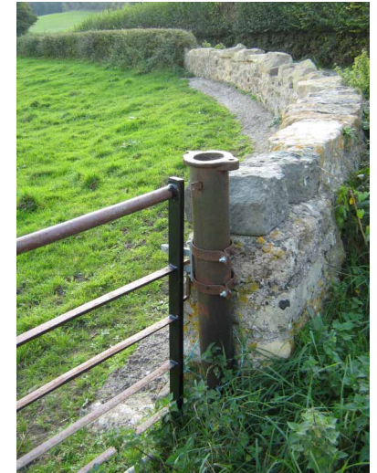
A 4-inch CAST IRON PIPE WITH COUPLING FLANGE PRESERVED AS A GATEPOST JUST BELOW THE ENGINE SITE
