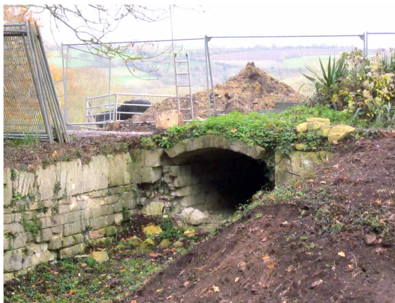
THE 'BOAT HOUSE' TUNNEL
