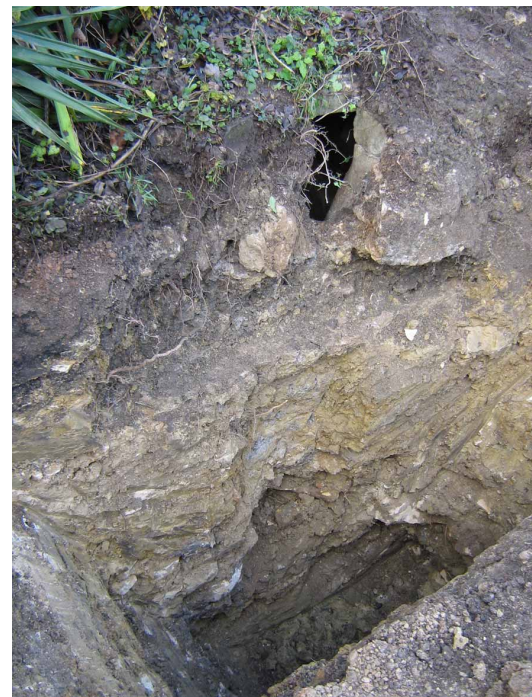
A 10ft. DEEP EXCAVATION TO REVEAL THE BACK OF THE TUNNEL (Site 3a) The rough face is the back wall of the tunnel. The hole is the top of a stone chute.
