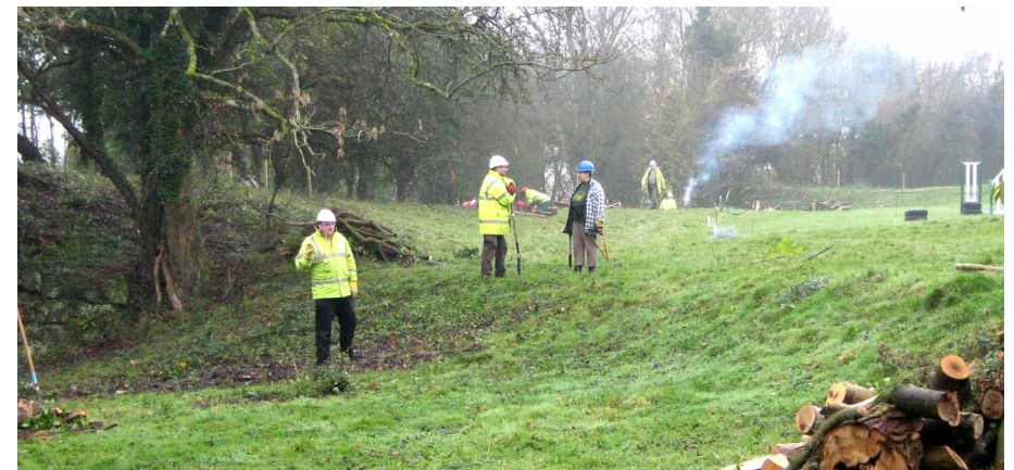
THE WATERWAY RECOVERY GROUP CLEARING LOCKS 2 TO 5
