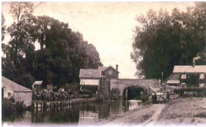
EASTINGTON WHARF ON THE STROUDWATER CANAL
