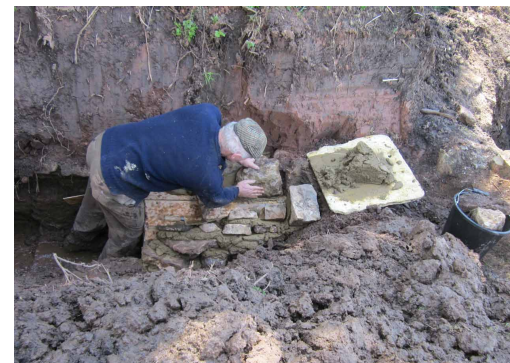
RICHARD HIGNETT REBUILDING THE CULVERT
