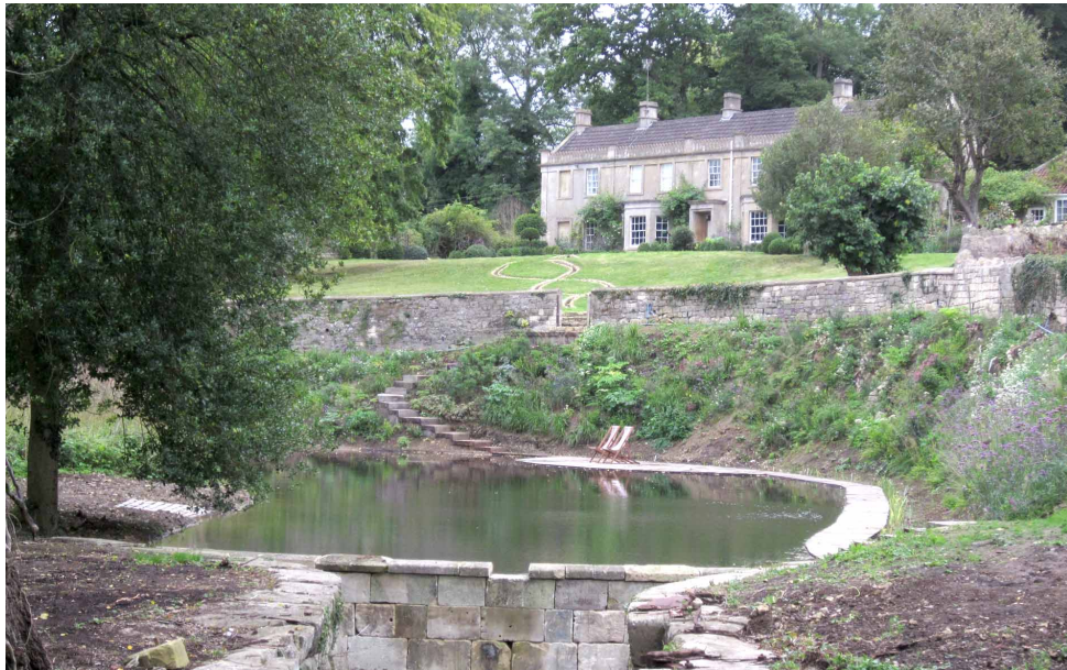
THE REFILLED POUND BETWEEN LOCKS 5 & 6 OF THE COMBE HAY FLIGHT with Caisson House in the Background
