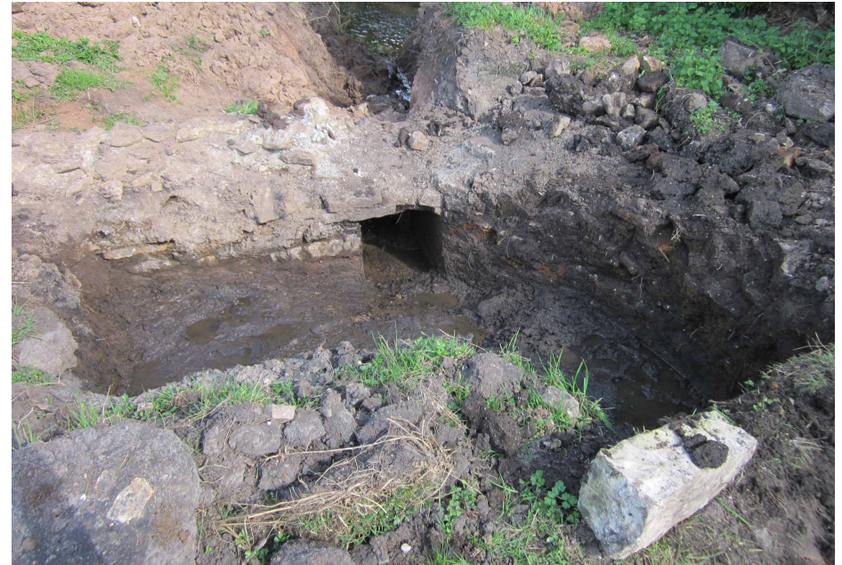
View 2 — THE SOUTH-EAST CORNER OF THE DRY DOCK showing the inside of the dock wall pierced by the drainage sluice. The wet (darker in appearance) area is the rough stone floor of the dock. A trench on the alignment of the culvert leading to the Cam Brook can be seen in the background.
