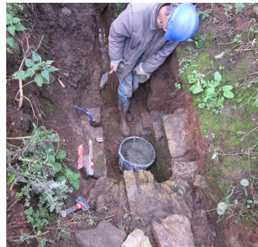
AERIAL VIEW OF REBUILDING THE DRY DOCK CULVERT
