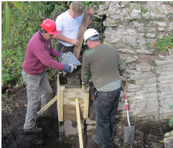
CASTING A NEW 'STONE' AT THE STOP PLANK POINT
