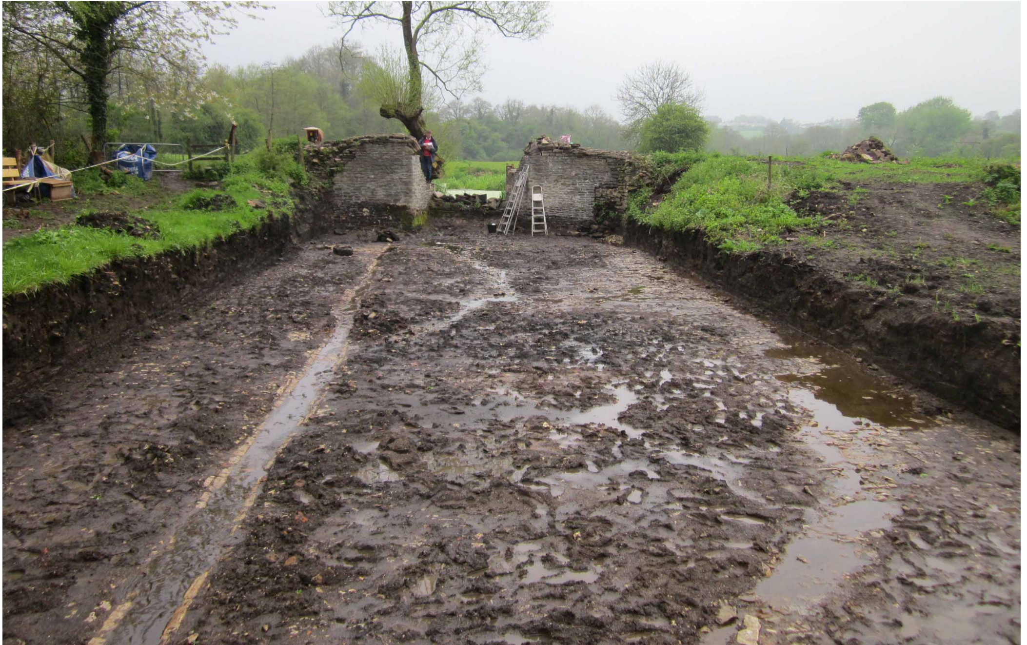
PAULTON DRY DOCK AFTER EXCAVATION
