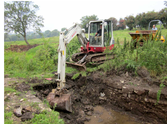
EXCAVATING TERMINUS BRIDGE
