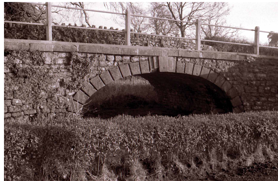
Photograph: Terry Paget VOBSTER CROSS BRIDGE OVER THE DORSET AND SOMERSET CANAL — 1959
