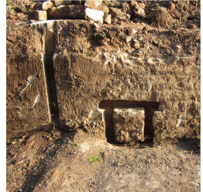
THE STOP PLANK GROOVE AND THE Π-SHAPED FEATURE AT WITHY MILLS NARROWS
