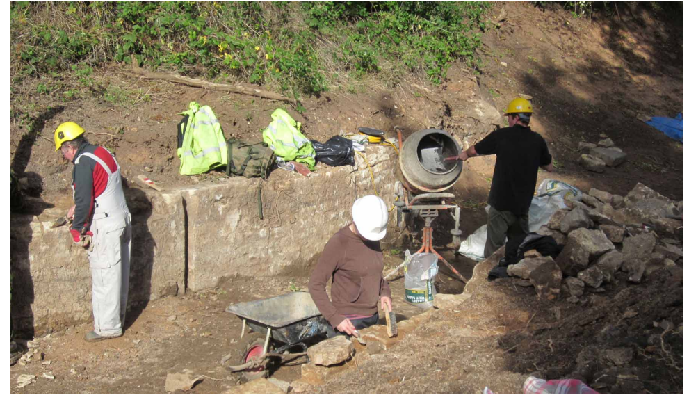
W.R.G. STONEMASONS REBUILDING WITHEY MILLS STOP POINT
