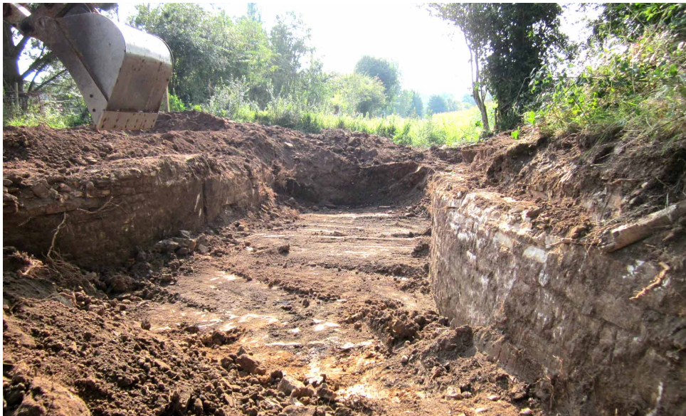
EXCAVATION AT WITHEY MILLS STOP POINT
