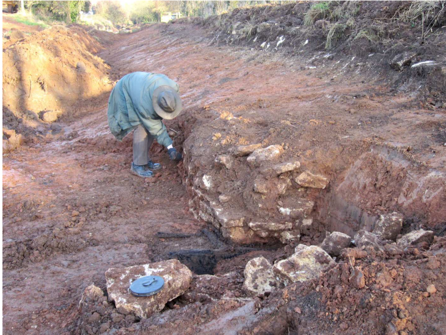
Above: MIKE CHAPMAN INVESTIGATING THE ROUGH STONE WALL WITH THE UNIDENTIFIED WOODEN OBJECT PROTRUDING FROM IT IN THE FOREGROUND (Some of the stones have been removed from the wall to investigate how far the object extends back under the embankment.)
