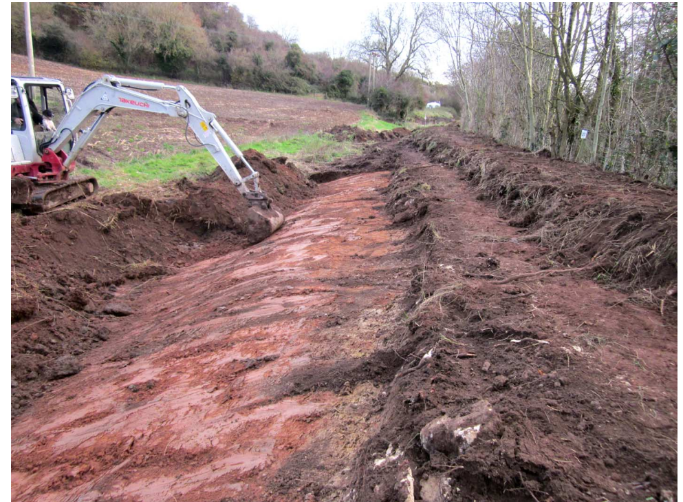
THE TOWPATH EMBANKMENT
