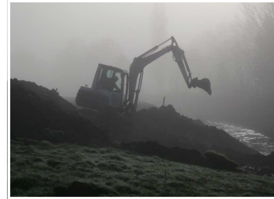
Above: DIGGING EARLY IN THE MORNING...
