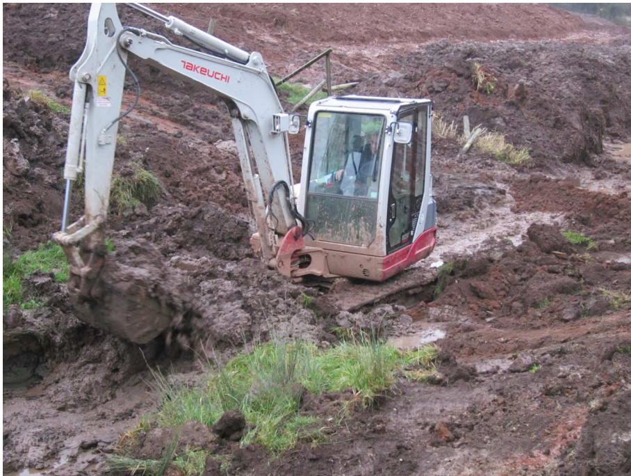
TIME TO GIVE UP — THE DIGGER COMPLETELY BOGGED DOWN IN MUD
