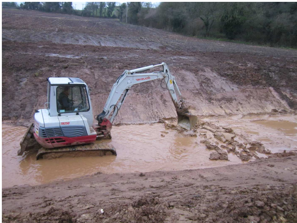
THE DIGGER PUDDLING THE CANAL BED
