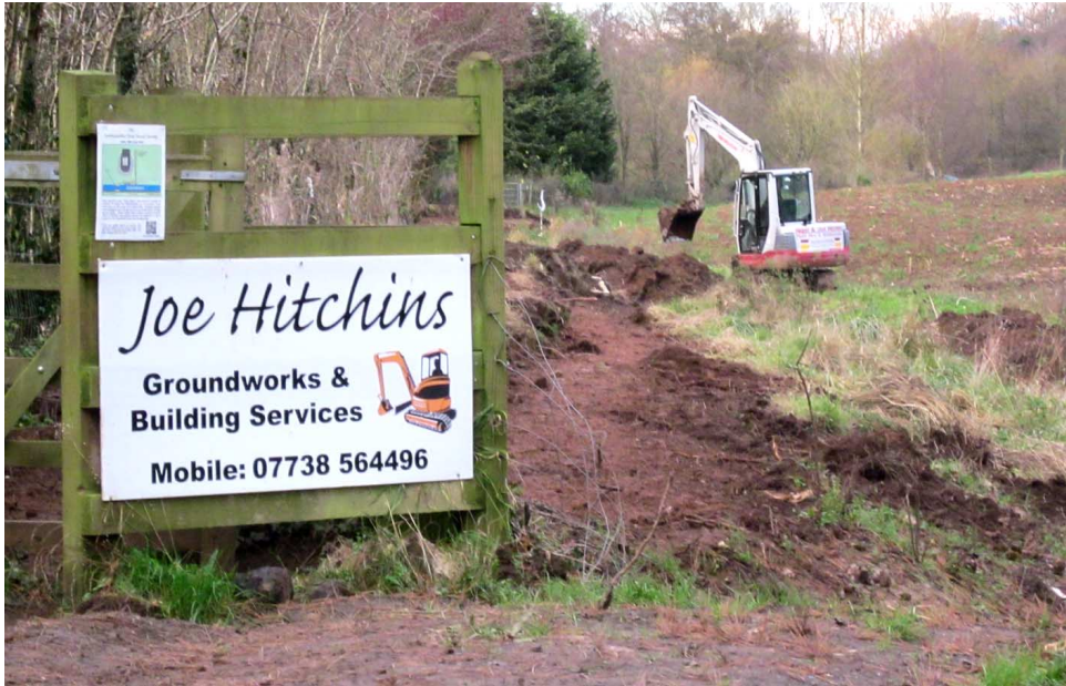
THE DIGGER BEGINS WORK ON THE TOWPATH WEST OF WITHY MILLS
