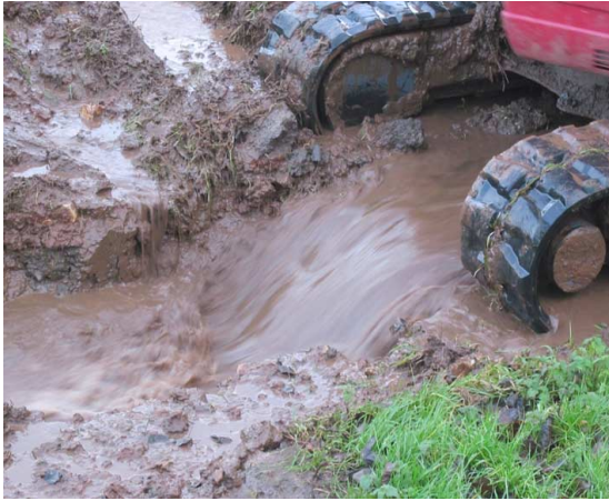
A DRAINAGE CHANNEL CUT BY THE DIGGER
