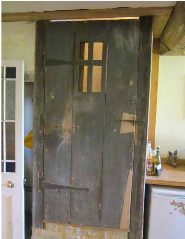
THE STAIRCASE DOOR INTO THE KITCHEN [Below]
