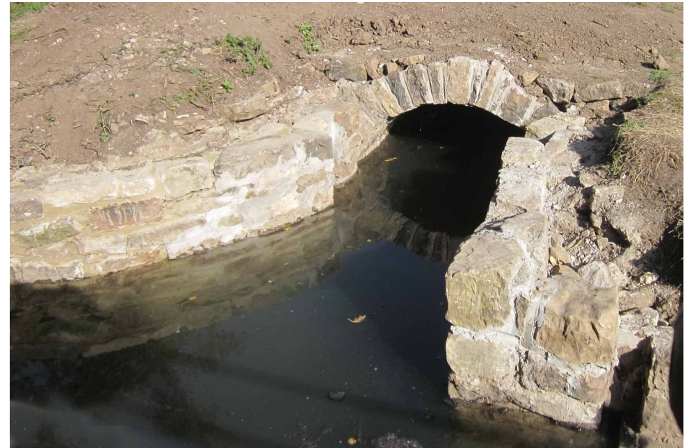
THE RESTORED OVERFLOW CHANNEL (Above) AND CULVERT (Below)
