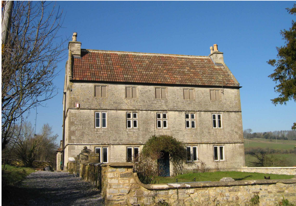
RUGBOURNE FARM HOUSE — 2008 before the attic windows were unblocked
