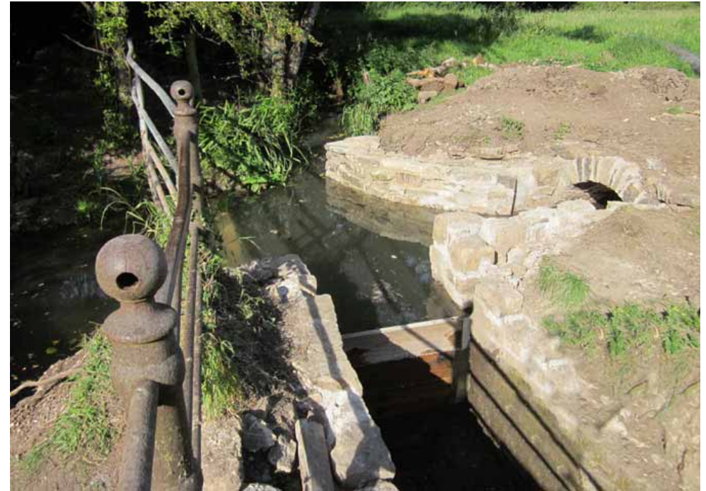
THE RESTORED OVERFLOW CHANNEL (Above) AND CULVERT (Below)
