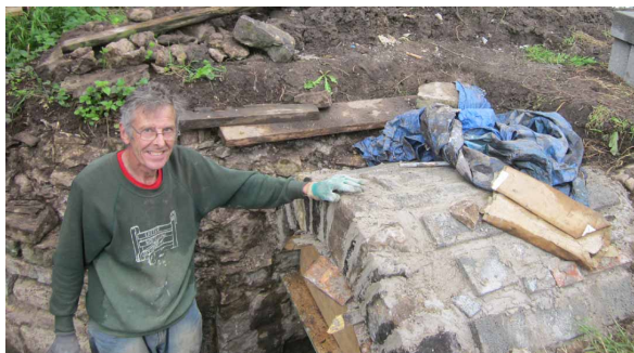
(Above) LIZ REBUILDING THE OVERFLOW CHANNEL (Below) ROB REBUILDING THE CULVERT ARCH
