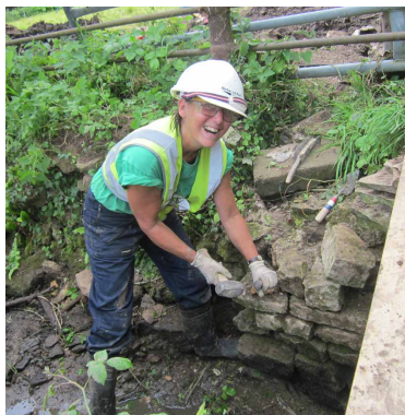
(Above) LIZ REBUILDING THE OVERFLOW CHANNEL (Below) ROB REBUILDING THE CULVERT ARCH
