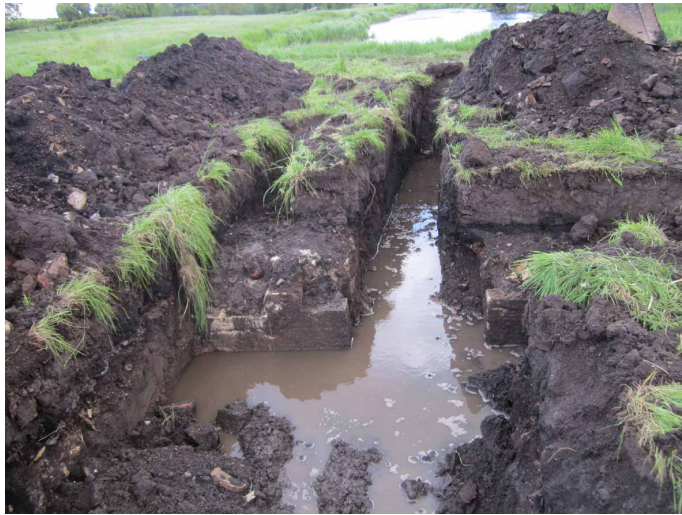
THE CHANNEL LEADING TO TIMSBURY BASIN THROUGH THE QUOINS OF THE RETAINING WALL
