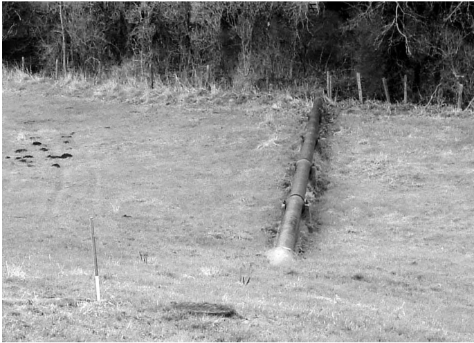
Fig.13 The capped shaft where the adit is joined by the pipe from Timsbury and the storm drain from High Littleton (the latter indicated by similar capped shafts in the next field to the left).
