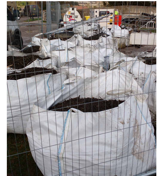
[Right] TONS OF REMOVED RUBBISH BEING STORED IN A TEMPORARY COMPOUND
