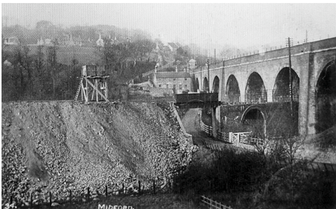
Fig. 4 — A VIEW OF THE BRIDGE OVER TWINHOE LANE, THE ARCH OVER THE CAM BROOK AND THE TRACKBED OF THE CAMERTON TO LIMPLEY STOKE LINE UNDER THE S&D RAILWAY VIADUCT AT MIDFORD.
