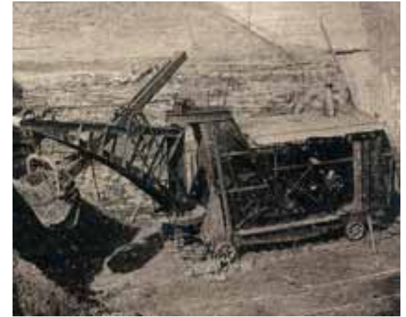
Fig. 12 — A DUNBAR & RUSTON STEAM NAVVY AT WORK ON THE MANCHESTER SHIP CANAL
