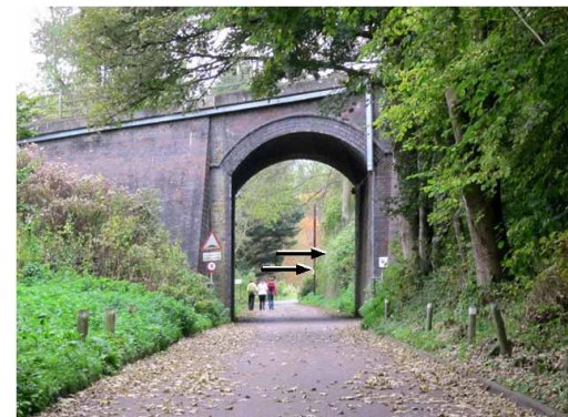
Fig. 7 — THE TRACKBED AT BRASSKNOCKER LOOKING WESTWARD THROUGH THE BRIDGE UNDER THE A36 ROAD
