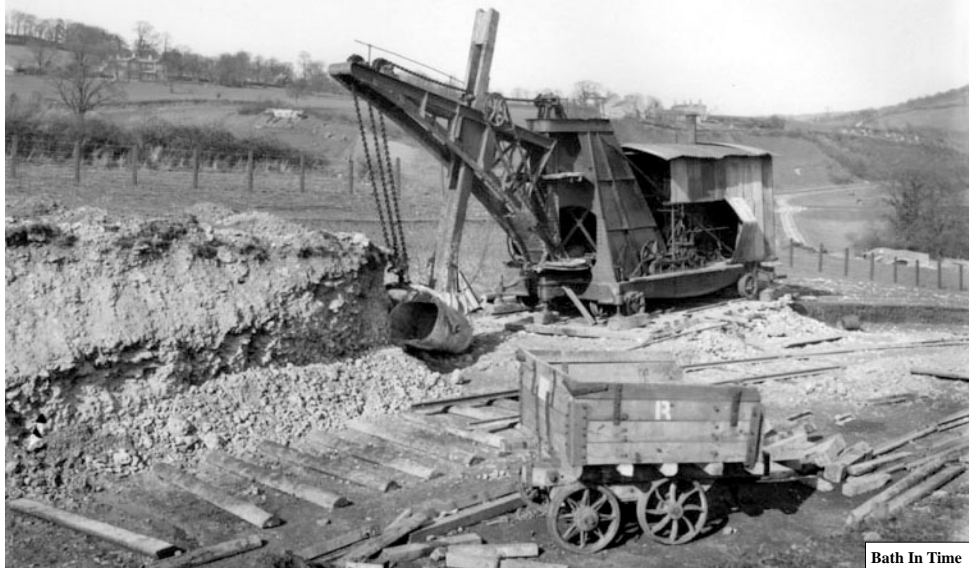
Fig. 11 — STEAM NAVVY ON THE UPPER MIDFORD EMBANKMENT
