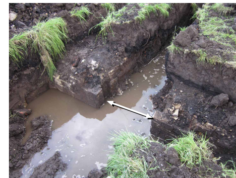
[Left] VIEW OF THE QUOINS SHOWING THE STOP PLANK GROOVES (arrowed).
