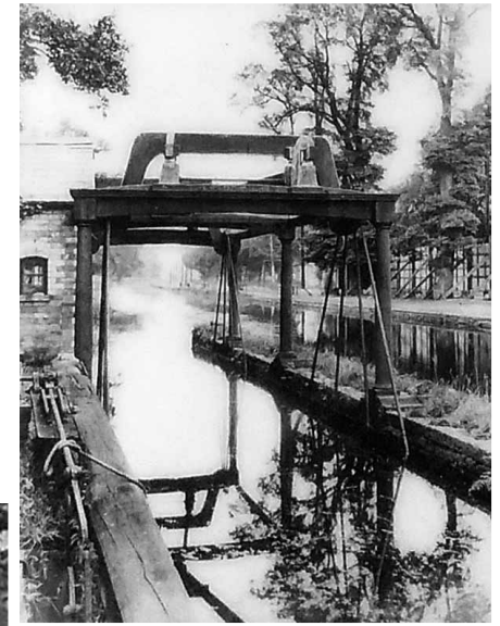
(Right and below:) TWO VIEWS OF THE WEIGHING MACHINE WHEN IT WAS INSTALLED AT NORTH ROAD, CARDIFF
