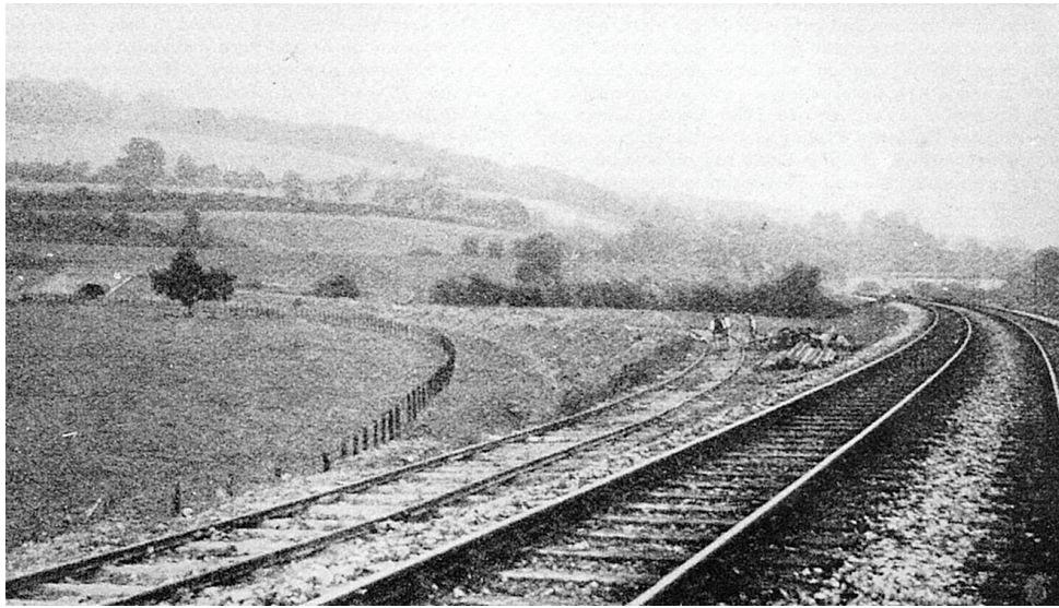
Fig. 15 — THE CONTRACTOR'S RAILWAY AND EMBANKMENT CURVING AWAY FROM THE MAIN LINE NEAR BRASSKNOCKER
