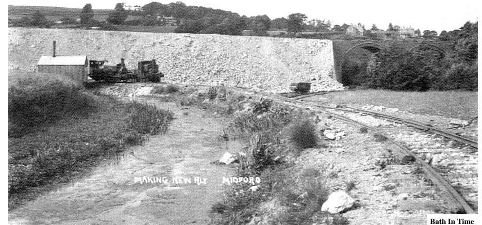
Fig 18 — UPPER MIDFORD EMBANKMENT LOOKING NORTHWARDS The embankment is nearly complete as far as Holley's Bridge. Note the two locomotives parked on the left branch line near the hut, the main line goes through the left (western) arch of Holley's Bridge and on to Midford.
