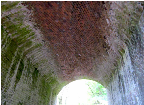
Fig 23 — SPIRAL BRICKWORK IN THE SKEWED ARCH OF MILLER'S BRIDGE
