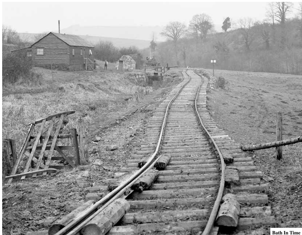
Fig 21 — THE CONTRACTOR'S RAILWAY AT LOCK 20 or 21
