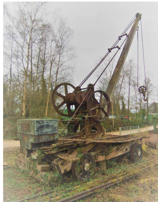
THE CRANE AT THE QUARRY SITE BEFORE RESTORATION
