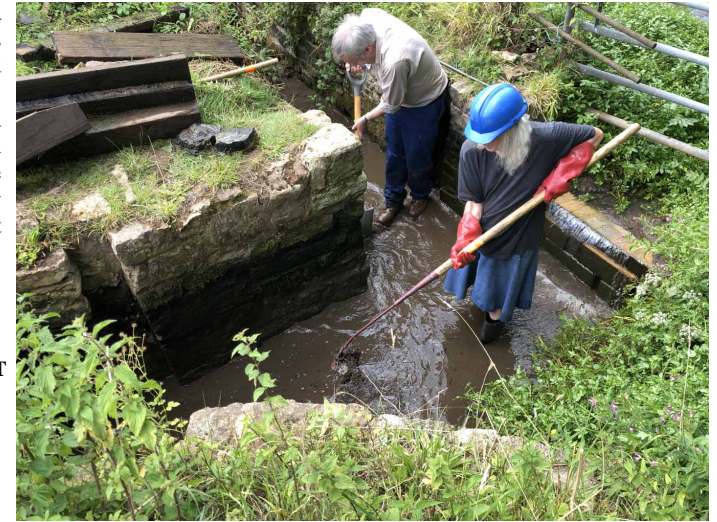
Right: JOHN DITCHAM AND LIZ CLEARING OUT THE SLUDGE TRAP
