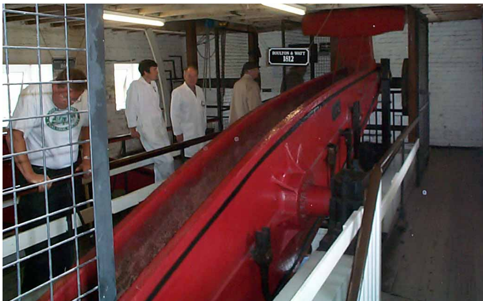
THE BEAM OF THE BOULTON & WATT PUMPING ENGINE AT CROFTON — July 2004 This is a contemporary of the Combe Hay engine which was later moved to Dunkerton. The beam is constructed from two iron castings with no wood involved.
