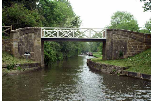
THE TYPE OF BRIDGE WE ARE PLANNING TO INSTALL AT PAULTON
