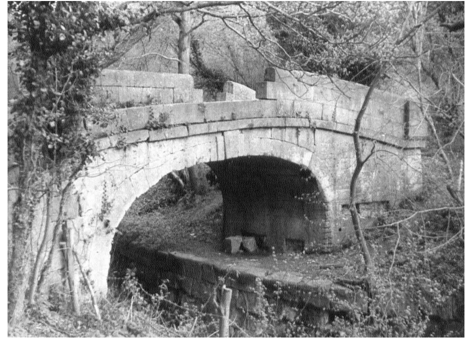
SOUTHSTOKE BRIDGE SHORTLY BEFORE DEMOLITION
