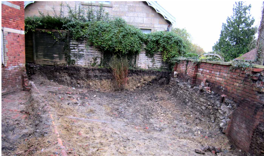
EXCAVATIONS AT RAILWAY LANE, WELLOW — November 2013 The profile of part of the canal bed is visible at the far end of the excavation
