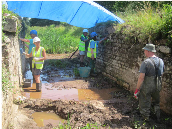
W.R.G./B.I.T.M. VOLUNTEERS RE-POINTING THE FOUNDATIONS OF TERMINUS BRIDGE
