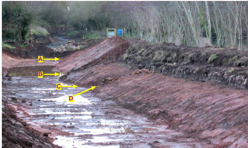
Fig 1 — EMBANKMENT PUDDLING UNDER CONSTRUCTION AT WITHY MILLS — December 2014
