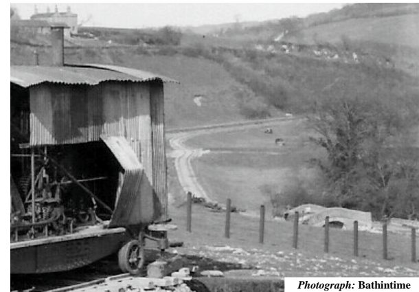
Fig. 9 — 'MAKING NEW RLY.' c1909 The temporary contractor's railway running along the former canal towpath towards the camera; past the entrance for the Midford Aqueduct (shown as a slight kink in the line) and towards the Midford Accommodation Bridge.
