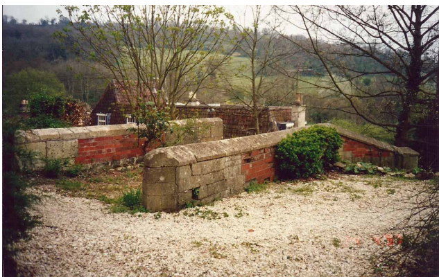
Fig 8 (Left) — TUCKING MILL BRIDGE — 1997
