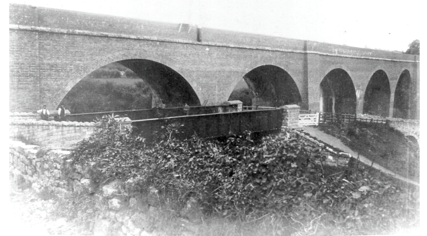
Photograph: S&DRT Fig. 14 — S&D RAILWAY VIADUCT & TWINHOE LANE BRIDGE c.1895 The 'New' Road Bridge over the canal.
