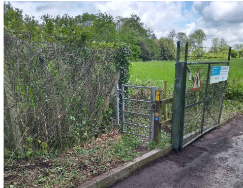
THE ENTRANCE TO THE COAL CANAL WAY CLEARED OF OBSTRUCTIONS
