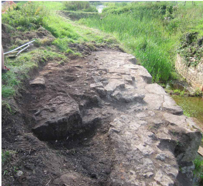
STONEWORK ON THE SOUTHERN ABUTMENT
