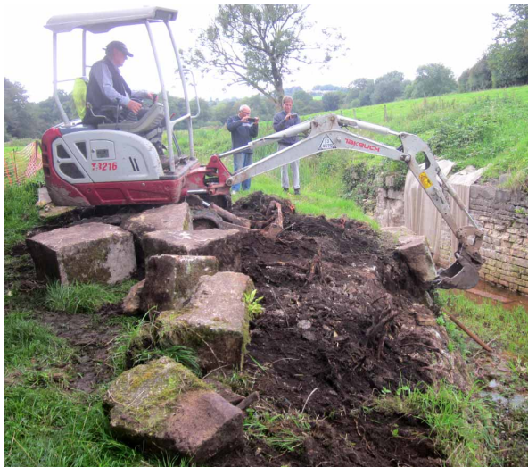
LARGE COPING STONES ON TOP OF THE WING WALL AT THE SOUTH-EAST CORNER
