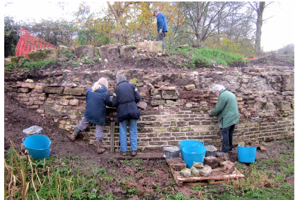
VOLUNTEERS REBUILDING THE WING WALL
