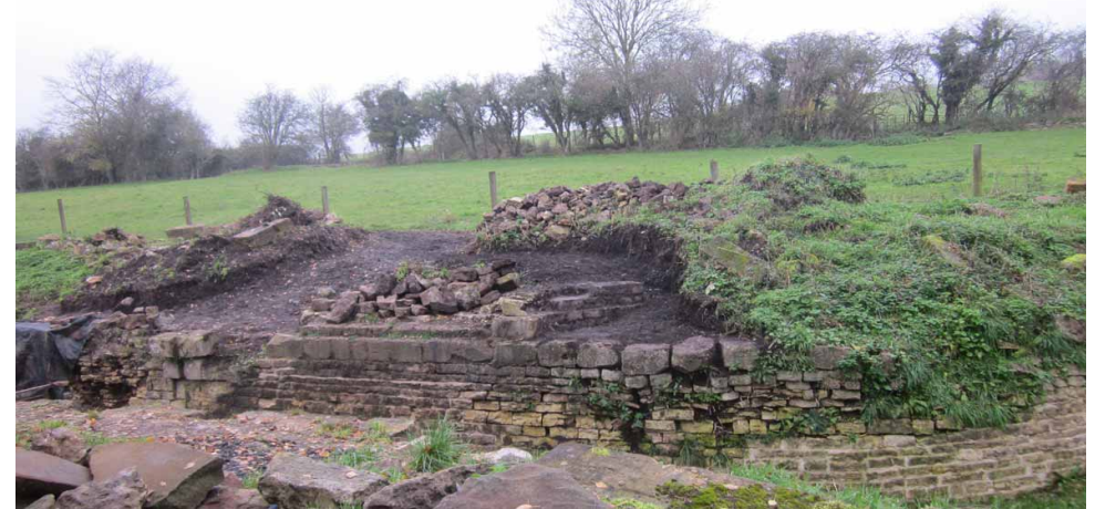
FOUNDATIONS COMING TO LIGHT ON THE NORTHERN ABUTMENT
