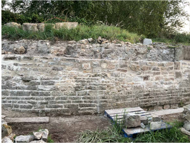
THE SOUTH-EASTERN WING WALL REBUILT TO COPING STONE LEVEL
