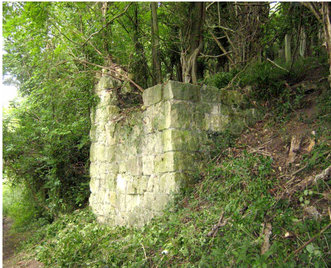
Fig.7 THE 'STAITHE' STRUCTURE ABOVE LOCK 19
