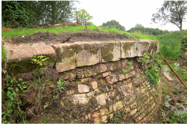
LARGE COPING STONES ON TOP OF THE WING WALL AT THE SOUTH-EAST CORNER
