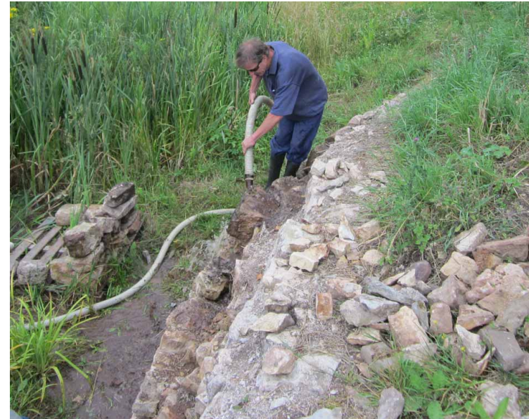
Left: JOSH GOULD WASHING OUT EARTH AND DEBRIS FROM THE DISMANTLED WALL
