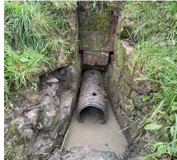
THE SLUICE OPENING WITH A TEMPORARY PIPE IN POSITION
