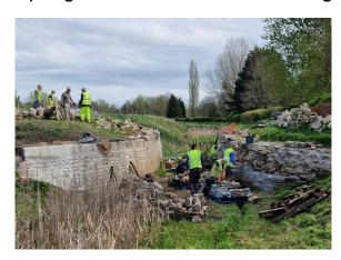
Immediately to the east of Paulton Basin Terminus Bridge allowed towing horses to cross the canal to reach Timsbury Basin. This bridge was also demolished many years ago but work party volunteers are currently rebuilding the abutment walls and an adjoining sluice so that the section of the canal in-water can be extended through this bridge opening into an already-excavated stretch of the canal.
